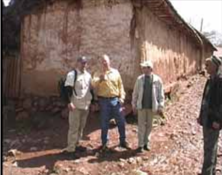
Poshum-This school is condemned. We are building a new school to open the door for evangelism next summer during the 2007 Campaign. Jeff Stamper (left above) gave his expertise to help plan the construction. Valerio (right) was amazed at the kindness
