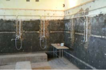
Showers being remodeled...
