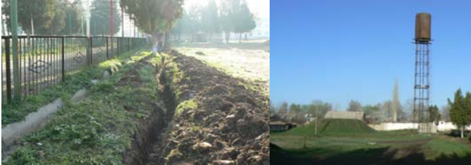
Left-Water line trench; Right-The small hill covers a 100 ton underground water storage tank next to the 60 foot water tower.
